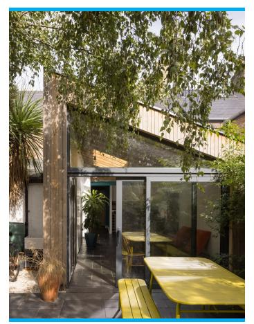
The Pitchglaze provides excellent thermal performance with a double-glazed specification featuring a laminated inner pane. The finish produces a smooth external look and being that the master bedroom looked down onto the pitched roof this was an important factor.
